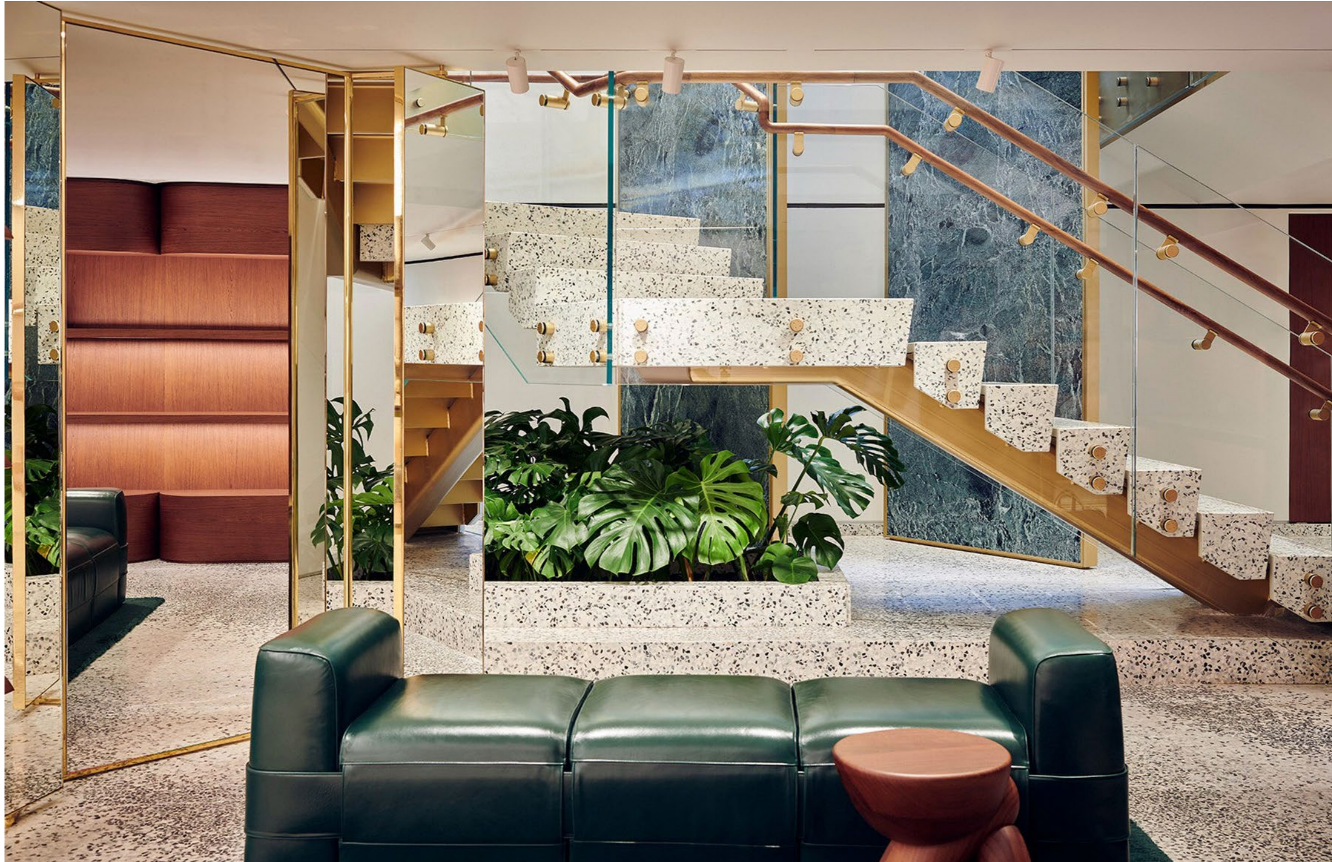
In London, the interior of a luxury boutique is elevated by a multi-material staircase with a steel load-bearing structure, Venetian terrazzo treads, glass balustrade, and wooden handrail.
